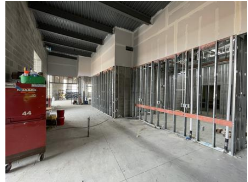
HS Office Drywall
