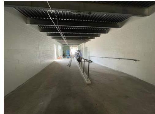
MS Ramp / Stairs
