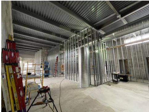
HS Office Framing
