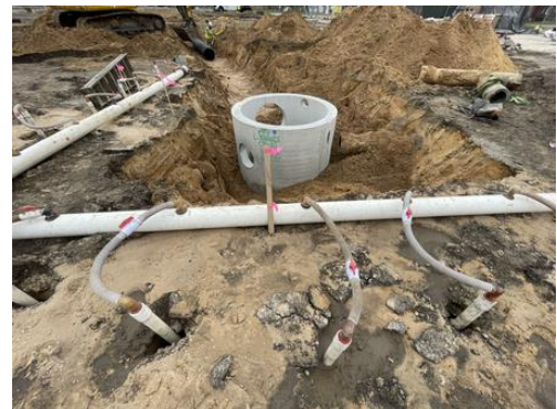
Dewatering for Storm Structures
