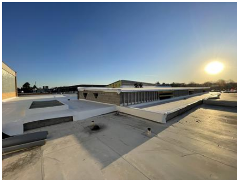
HS Office Roof
